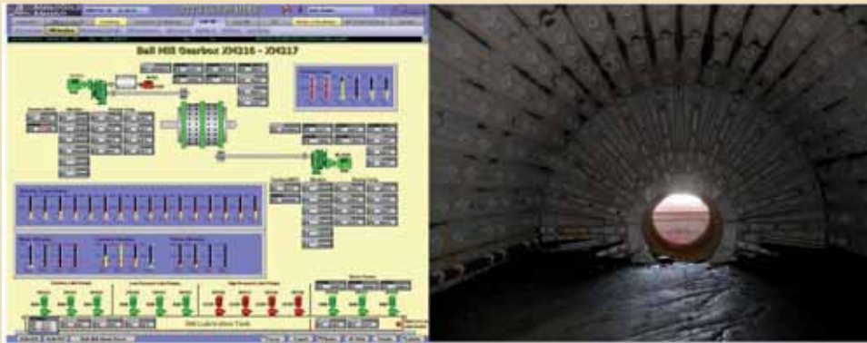
Figure 2: InTouch HMI screen showing a ball mill gearbox's lubrication details (left) and the view from inside the ball mill powered by the two 4MW motors shown in the graphic.
